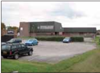
02 Existing Photo View from The Crab Apple public house car park
