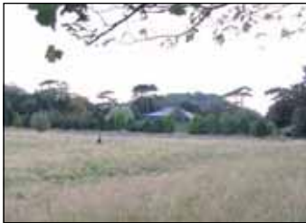
03 Existing Photo View over site, including disused tennis courts and former St Brandons Junior School buildings
